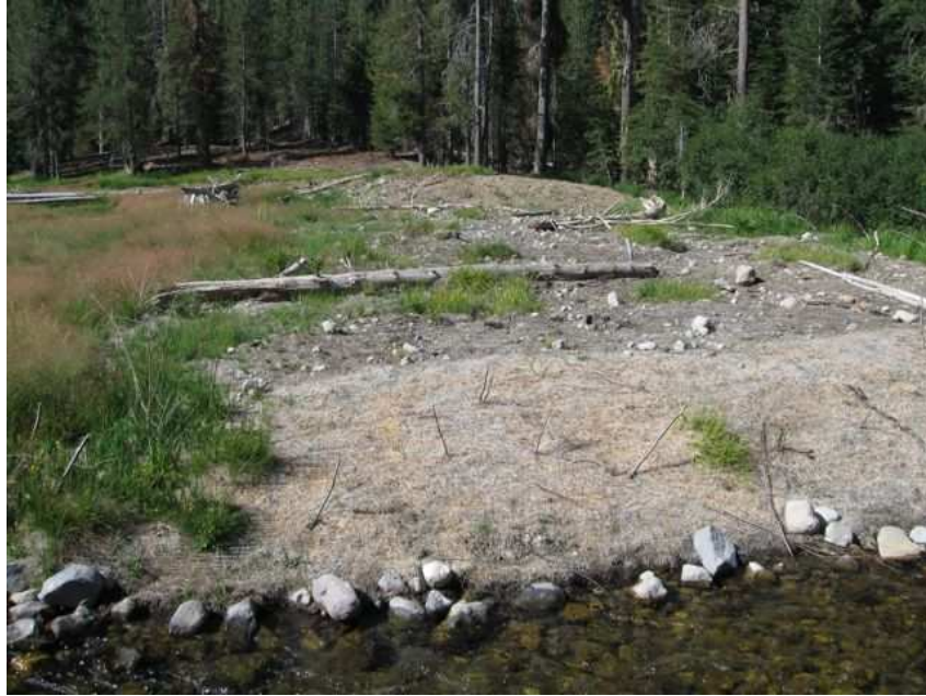
Fig. 3. Photo of Dream Lake Dam, following removal and leveling. Outflow channel in foreground was created by NPS during drawdown and draining of the lake in August of 2011.
