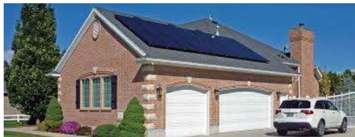
**Figure 7: Asphalt Shingle with Solar Panel System**
