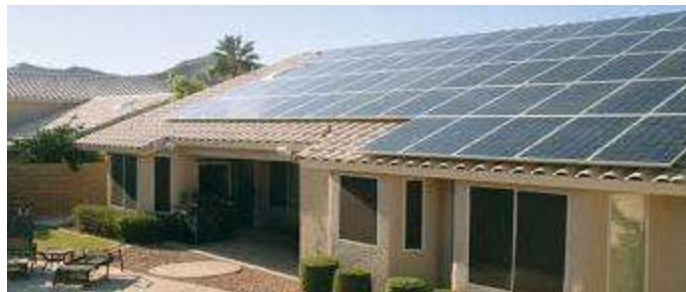
Figure 6: Ceramic Tiles with Solar Panel System
