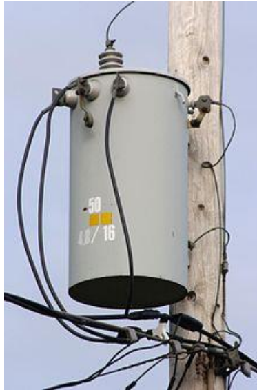
Fig. 1: Typical pole mounted distribution transformer [3]
