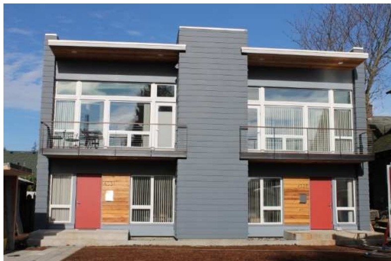
Figure 2-3 Trekhaus, a passive house duplex home, is divided into two mirror-image apartments with a party wall on the north-south axis. on the southern wall, total floor area, infiltration rates, ventilation rates, and envelope construction. The model in this simulation study is a single floor and a stand-alone structure. The building has a conditioned floor area of 148.6 m 2 , and
