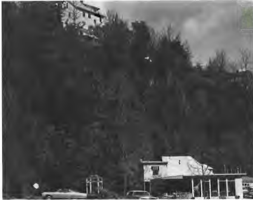
Figure 3. Photo of fairly secure site; cliff is bedrock rather than soil.
