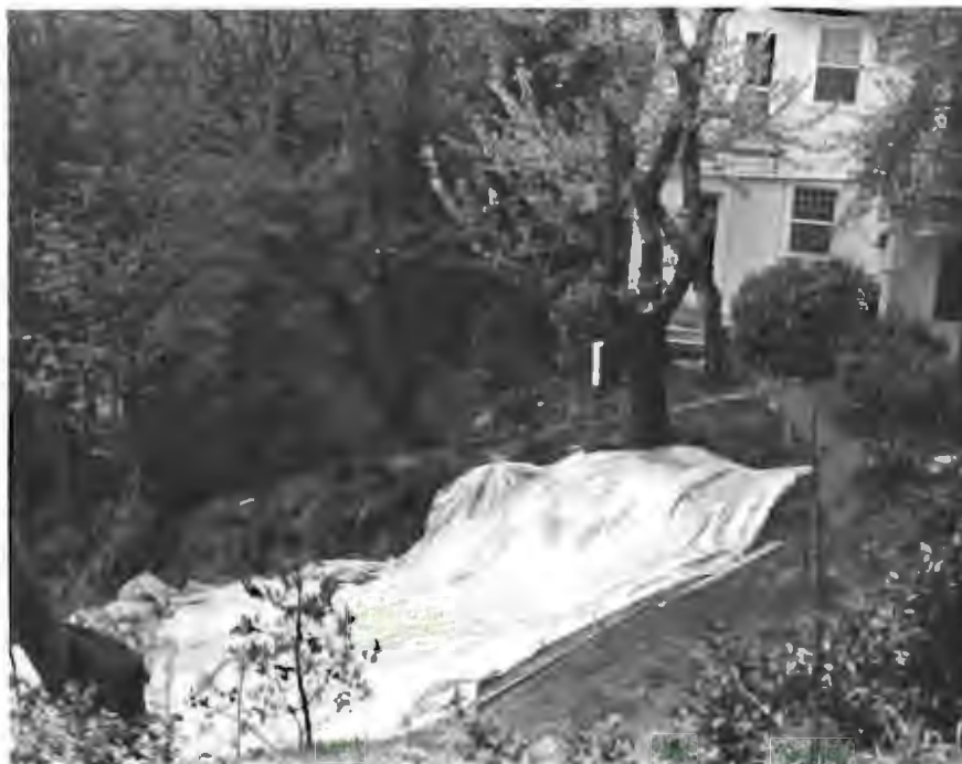
Figure 6. Photo of hazardous building site; a landslide scarp.
