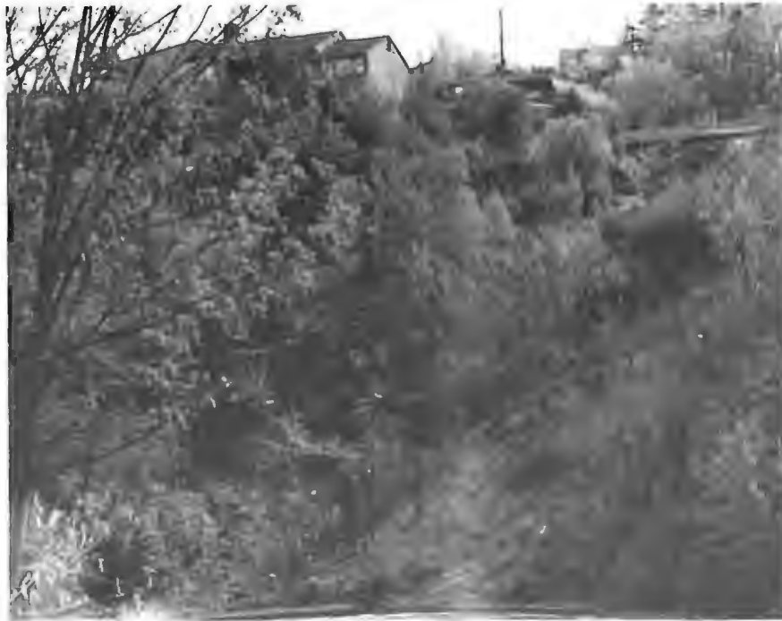
Figure 5. Photo of a poor building site; steep slope, lack of older permanent vegetation, and drainage course.
