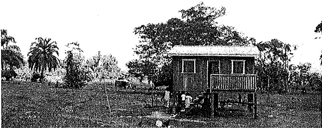
Figure 16. Traditional house with tin roof
