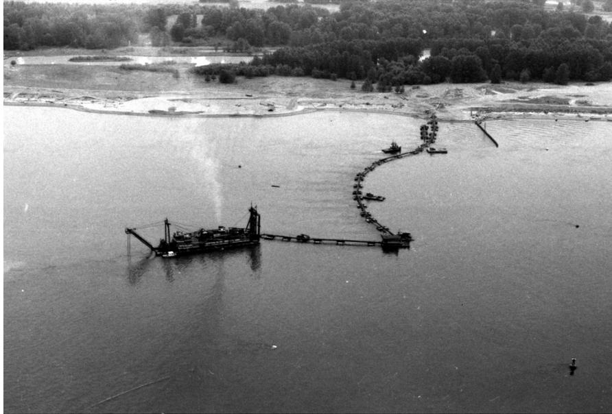
Figure 17. Dredging near Longview, Washington in response to Mount St. Helens eruption. Material is removed from the river bottom, transported through a pipeline, and deposited on land. U.S. Geological Survey photo taken by R. Schuster on July 10, 1980.
