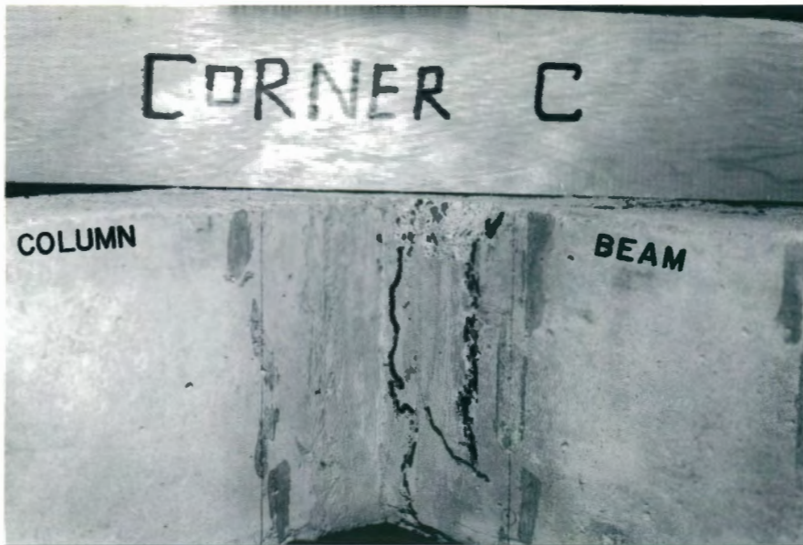
Fig. 5.13. Concrete spalling at corner C
