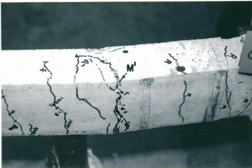
Fig. 5.28. Flexural-shear crack at M' (positive moment cutoff point)
