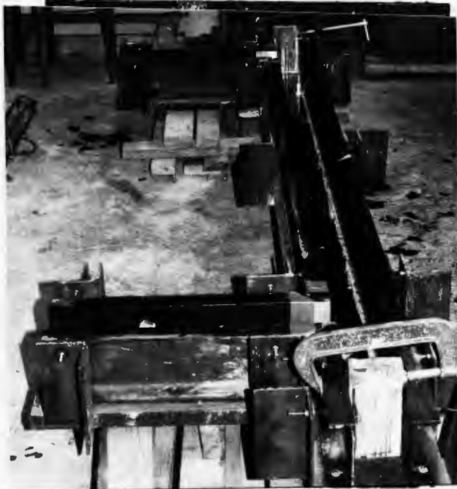
Figure 3.4. Form preparation before placing beam and column cages
