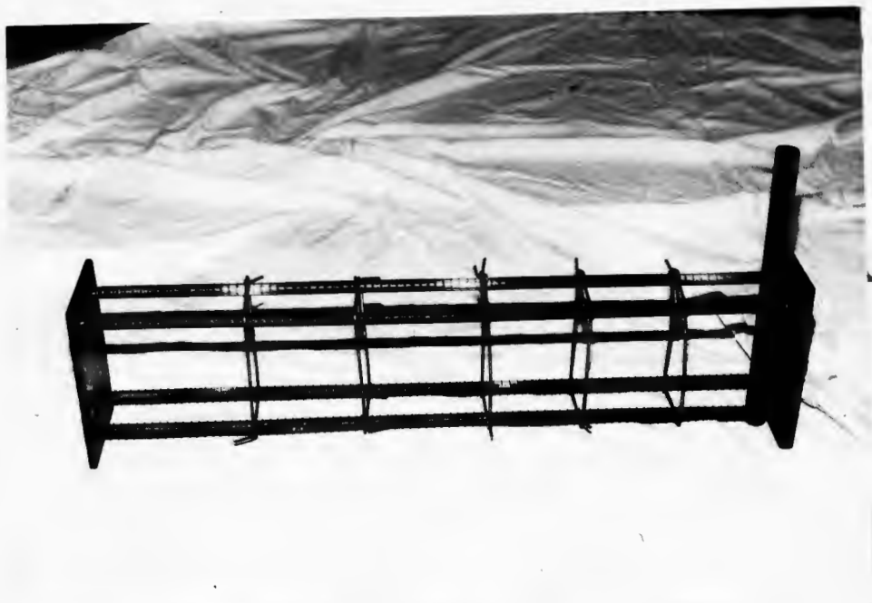
Figure 3.5. Column cage assembly
