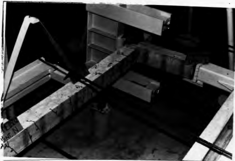
(b) CRACKS AT THE BEAM
