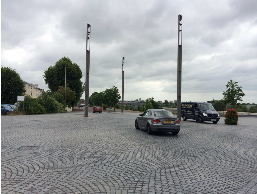
Figure 9: Elwick Square with the light posts, planters, and textured paving
