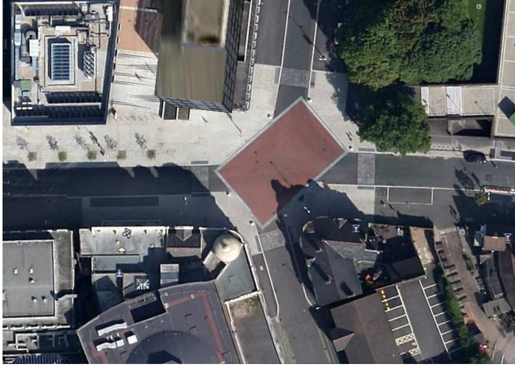
Figure 18: Aerial view of Coventry intersection (google.com, 2015)
