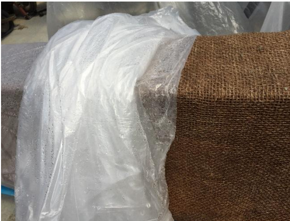
(E) Concrete condition after 12 hours of covering – still wet
