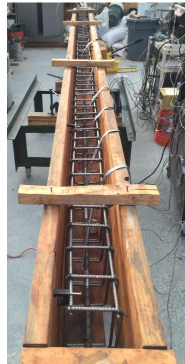
(B) Steel cage inside the wood frame
