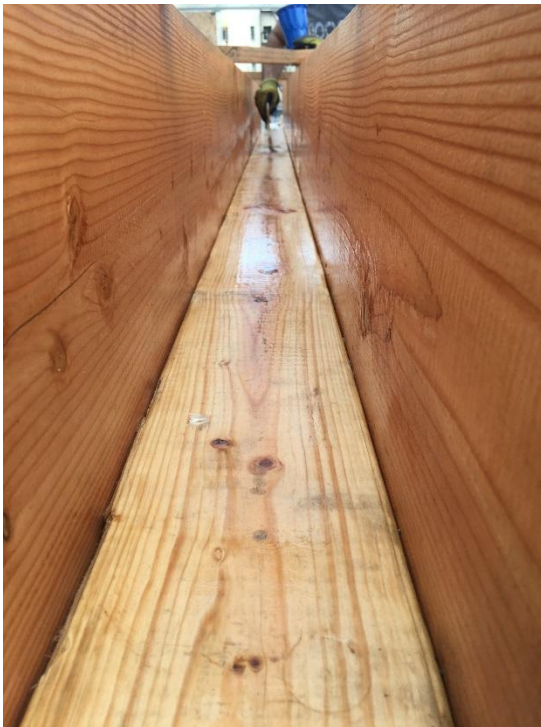
(A) Formwork/ oiling the interior surfaces.
