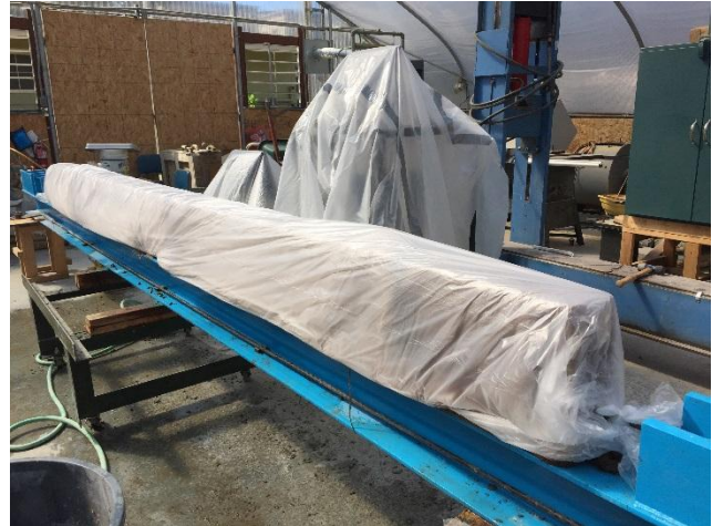
(J) Plastic covers in addition to the wet burlap
