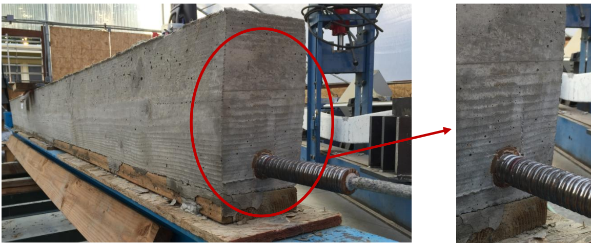
Figure 4.8 Typical view for Beam #4 showing the anchoring technique of CFRP strand at the ends.
