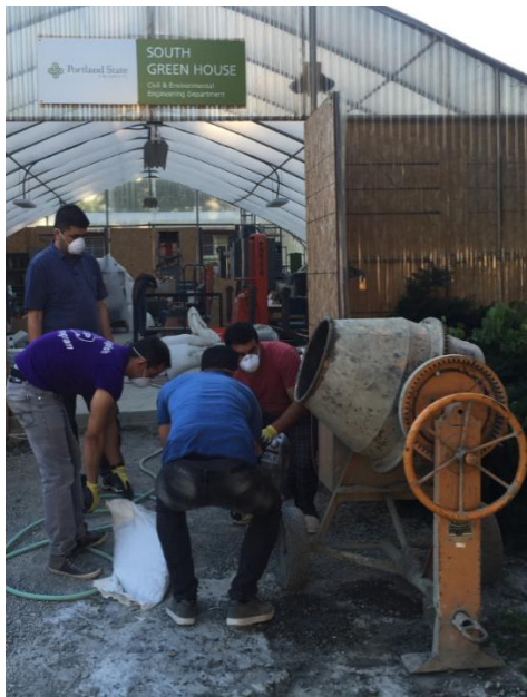
(E) Mixing concrete
