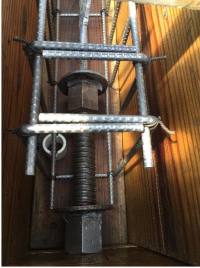
(C) The end anchors for Beam #4
