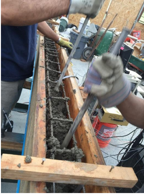
(E) Compaction using steel rods
