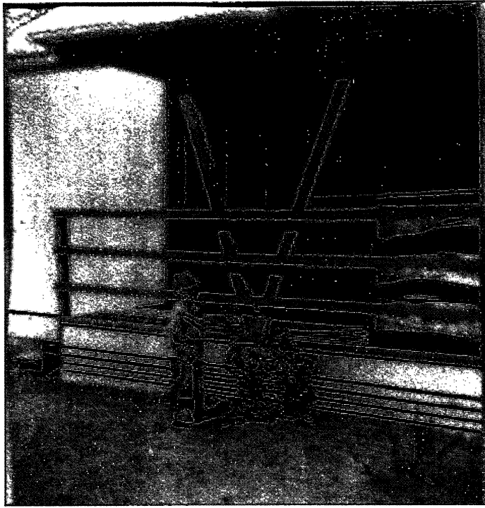
Figure 4-9. (photo) Porch of a duplex electric unit showing the “V for Victory” support beams. Courtesy of William Wier Hillgaertner.
