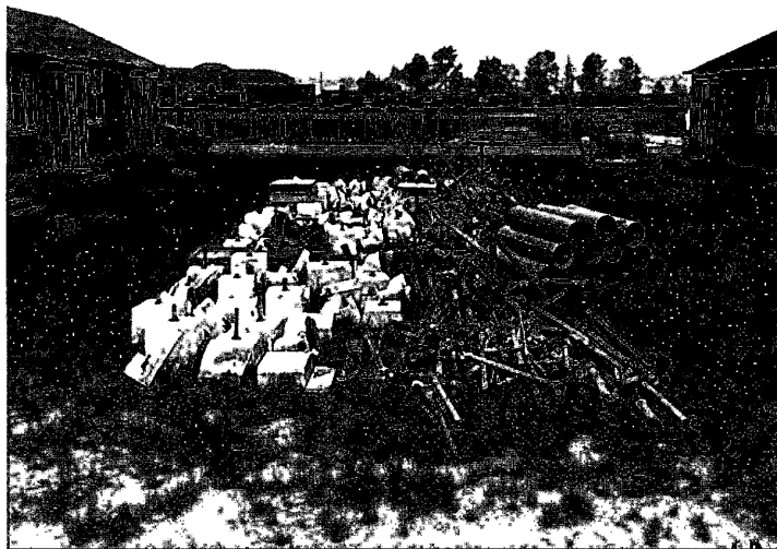
Figure 9-2. (photo) Salvage pile of sinks, pipes, and water heaters from dismantled Guild's Lake Courts units in 1946. Location not given on back of photograph. These are units from 44th Court because only the African American section had a fence and because of the proximity of the railroad to the units. The siding on these units appears to be thick paper over gypsum board. Courtesy of the City of Portland Archives, A2001.
