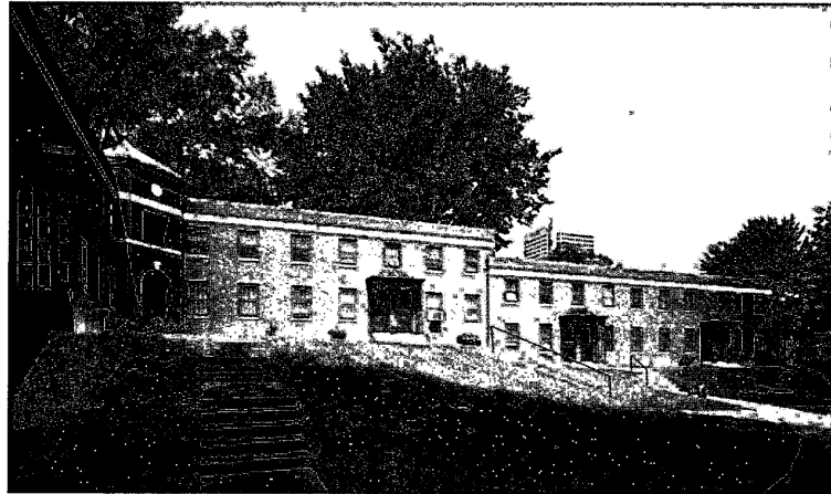
Figure 3-3. (photo) A few of the dwelling units at Techwood Homes, Atlanta, Georgia, prior to their demolition in 1996. Building Number 16, 488-514 Techwood Drive, these homes were the first federally funded demonstration public housing project to start construction. Courtesy of Library of Congress Prints and Photographs Division, Historic American Buildings Survey or Historic American Engineering Record (HABS GA,61-ATLA,60S-).
