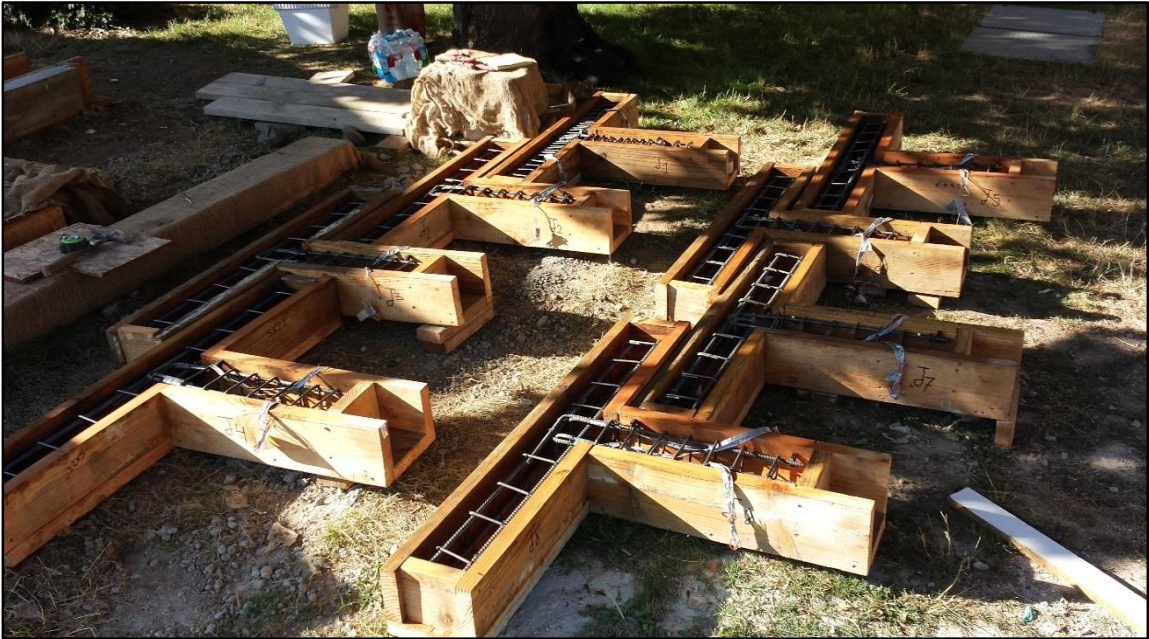
a- Preparing the molds for casting
