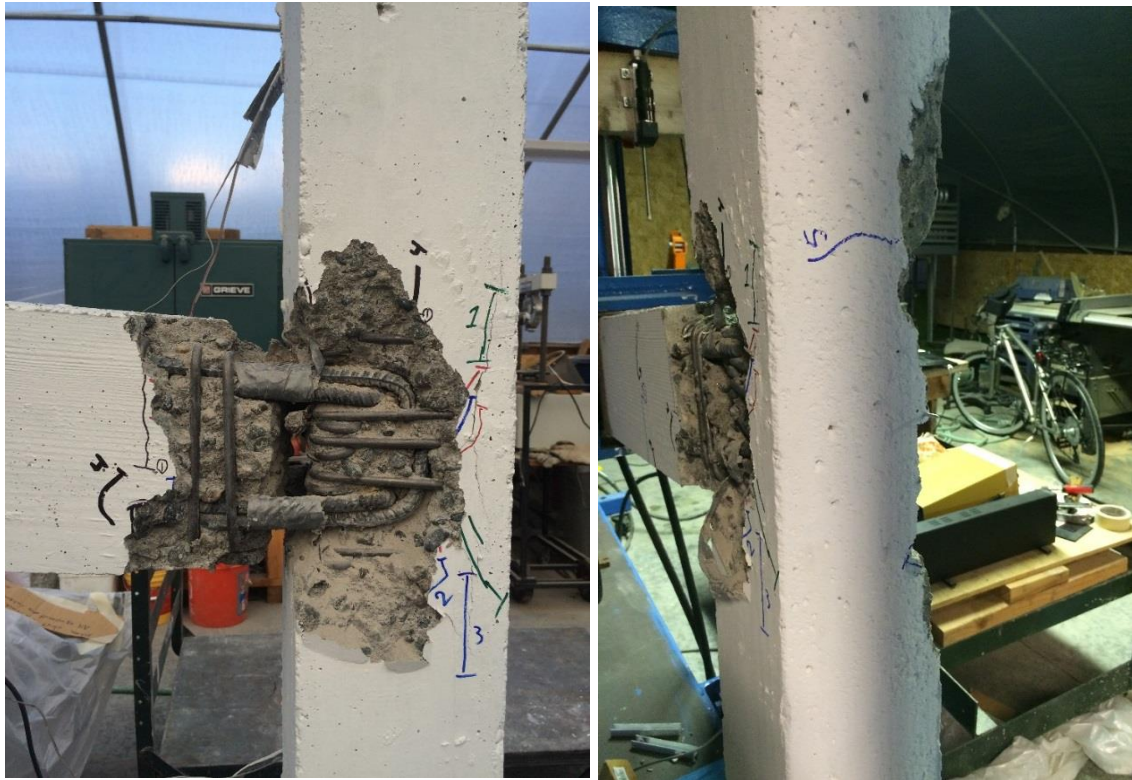
Figure 4-8 Specimen J1 (final crack pattern)
