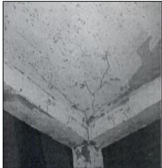
b- Beam-Column Joint with Slab
