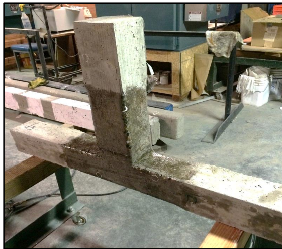
Figure 3-23 Applying the Prime Layer to the Concrete Surface
