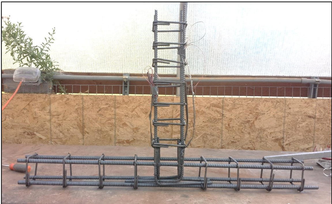
Figure 3-10 Reinforcement Cage of Specimen J2
