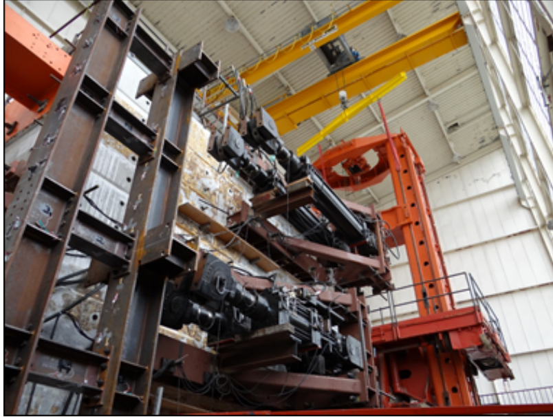
Figure 5.19: Actuator brackets installed on the reaction wall.
