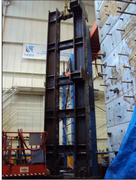
Figure 5.12: Linked columns of LCF-5L specimen being installed on the LC floor beam.
