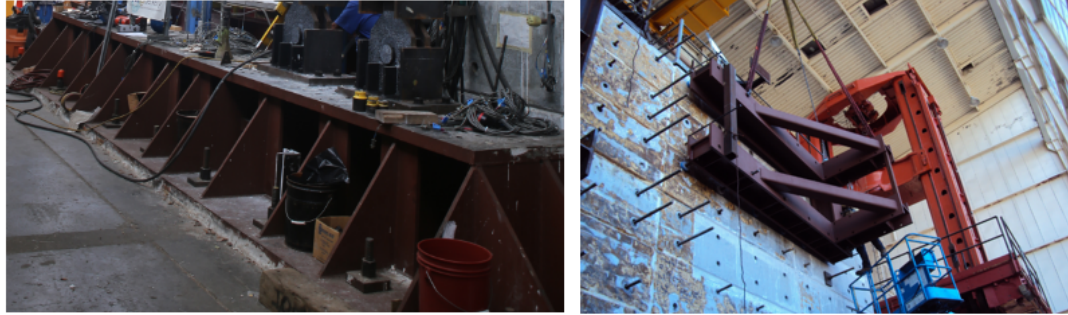
(a) LC floor beam
