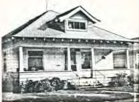
House with hip roof.
