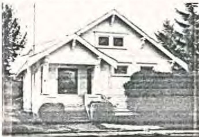
1015 North Galloway Street
