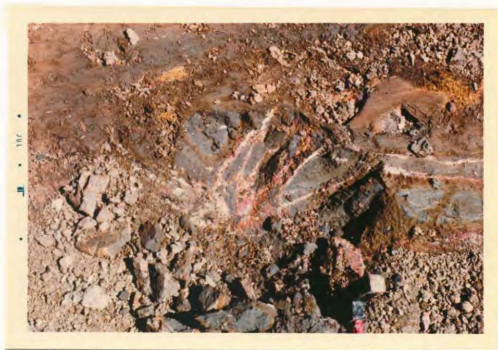
Figure 18. Clay-filled fractures in basaltic corestone from the high MgO flow of the Turner Freeway profile.
