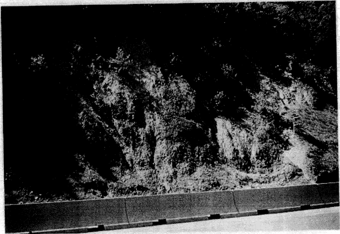
Figure 27. Photograph of fracture zone east of the weigh station. The zone is approximately 15 meters wide.
