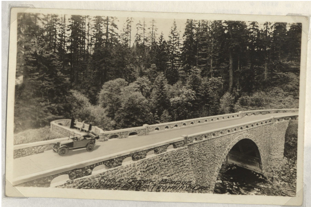
Figure 14 Bridge across Eagle Creek on the Columbia River Highway, c. 1916. Gerald W. Williams Collection, OSU SCARC.
