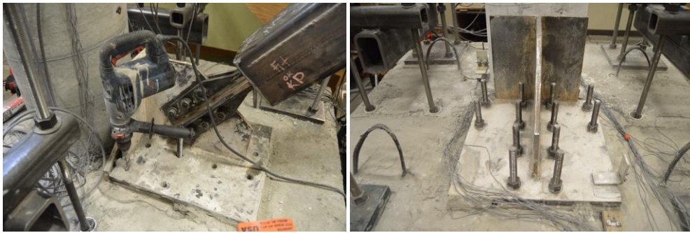
Figure 5.20 Post-installed anchors for gusset plates
