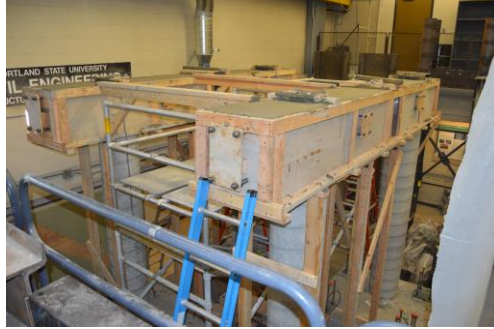
Figure 5.19 Construction sequence of RC bents
