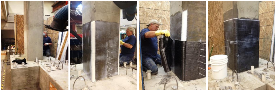
Figure 3.7 Installation of composite jacketing on a seismically deficient RC column
