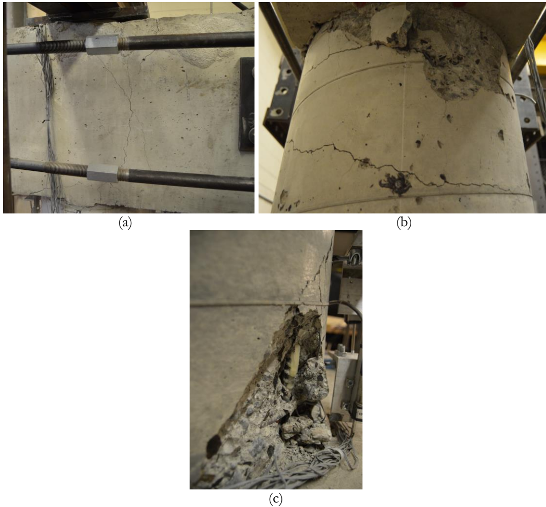
Figure 5.57 Damage in As-built Bent 2; (a) Damage in cap beam, (c) Significant spalling in columns, (c) Onset of rebar buckling
