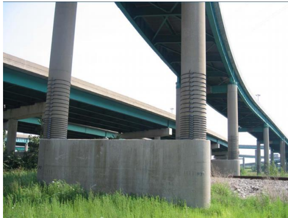
Figure 3.9 External prestressing steel retrofitting of columns in Illinois.
