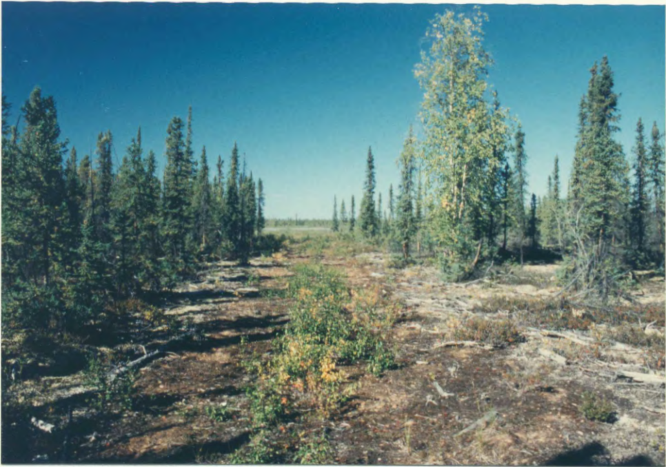
Figure 18. Roadway illustrating the general absence of vegetation, particularly shrubs, in the track areas after 10 years of abandonment. This is attributed to the destruction of near-surface rootstocks and vegetative propagules. Trees in the adjacent control average 3.5 m in height (Site # 8).
