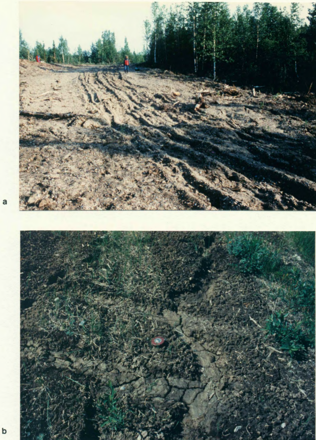
Figure 13. Surface rutting. a) on a sloping roadway section ( 4^{\circ} ), constructed by "cut -and - fill" practices in glaciofluvial gravels during the previous winter. The rutting was due to passage of vehicles too late in the spring (Site #2); b) hydraulic erosion caused by the unseasonal passage of All-Terrain-Vehicles on the right-of-way (Site # 1). Note the frothy appearance of the soil as a result of needle-ice formation.
