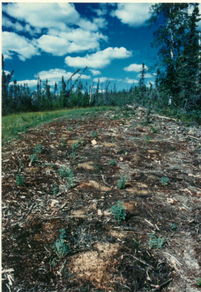
Figure 12. Scuffed earth hummocks. Note book for scale. The road shoulder has been cleared to a width of 6 m to enhance visibility in a road bend (Site # 1). Peat layers are preserved at 10 - 15 cm and inhibit revegetation due to summer drought. The grass-covered roadway, on the left, has been in operation for at least the past 18 years. Trees in the adjacent control average 6.5 m in height.
