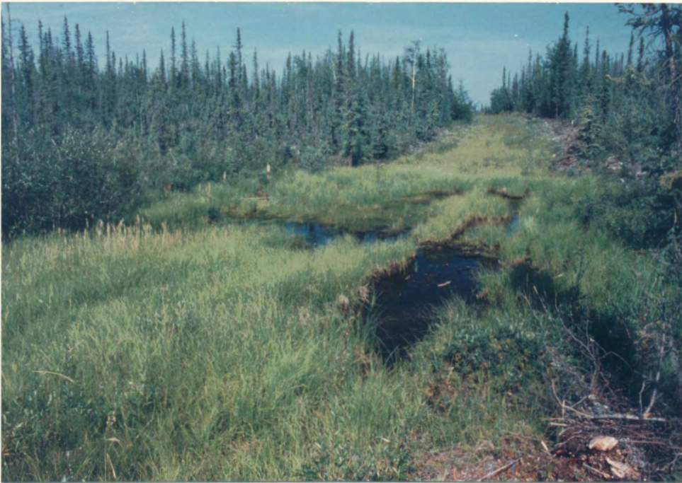
Figure 10. Ground subsidence on right-of-ways. a) uniform thaw settlement in excess of 1 m due to thawing of supersaturated sediments (Site # 3); b) differential thaw settlement (Site # 3) resulting from the thaw of ice wedges. Water is impounded in vehicle tracks and the thaw depressions. Black spruce in the adjacent control averages 3.5 m in height. Roadway vegetation dominated by sedges and grasses.
