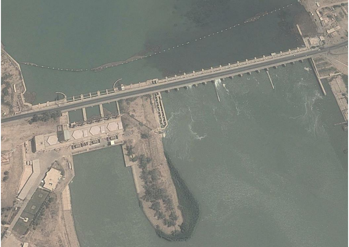
Figure 6: Samarra Barrage (Google Earth).
