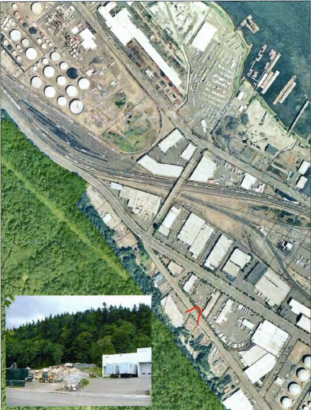
Figure 20: The aerial photo shows the intersection of Highway 30 and St. Helens Rd. The North Pacific Railyard can be seen next to Chevron and Phillips refinery storage facilities in the upper left corner of the image. Taxlot lines overlay the photo and Forest Park is shaded green. Inset photo, taken by Author, shows a wood pallet depot that abuts the park boundary on St. Helens Rd. Many businesses on St. Helens Rd. transfer or use hazardous and flammable materials, including fueling stations, fuel distribution and storage. (Source: air-photo courtesy of Spencer B. Gross, Inc.)
