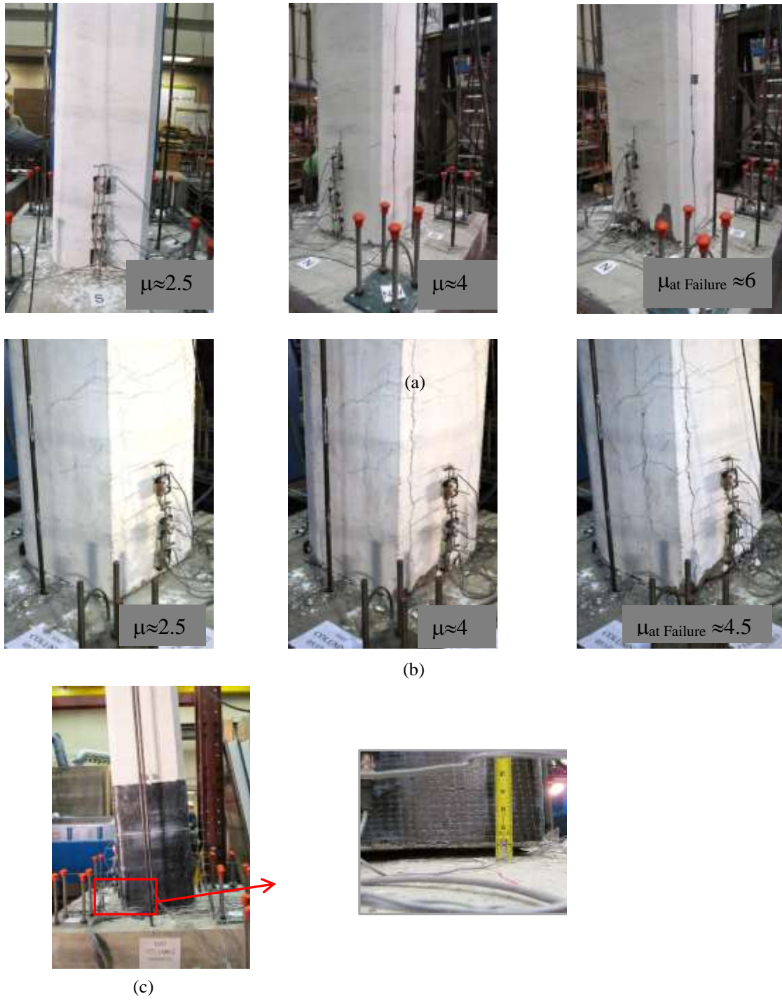
Figure 4-16 Observed Damage (a) A-C; (b) A-S; (c) R-S
