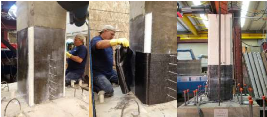
Figure 4-13 CFRP Retrofit Application
