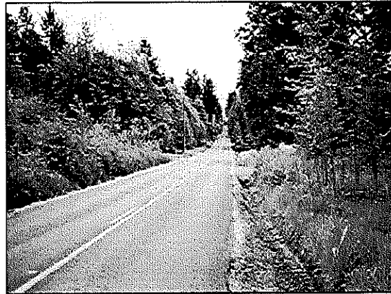
Figure F.2. DVA model visibility factors. 1) short in-line visibility, high road sinuosity, 2) long in-line visibility, high vehicle speeds, 3) dense vegetation adjacent to road hides approaching deer.
