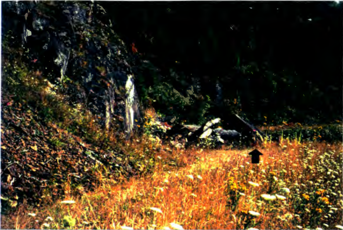
Figure 25. Slab block failure in a fragmental igneous unit - FS Rd. 310, ctr. sec. 16, T.5 N. R.5 E. Large failure blocks are common in the more welded ashflow units, which have jointing habits more similar to compact igneous bedrock. These slabs are as much as 4.7 m in length. Backpack (arrow) is .3 m for scale.
