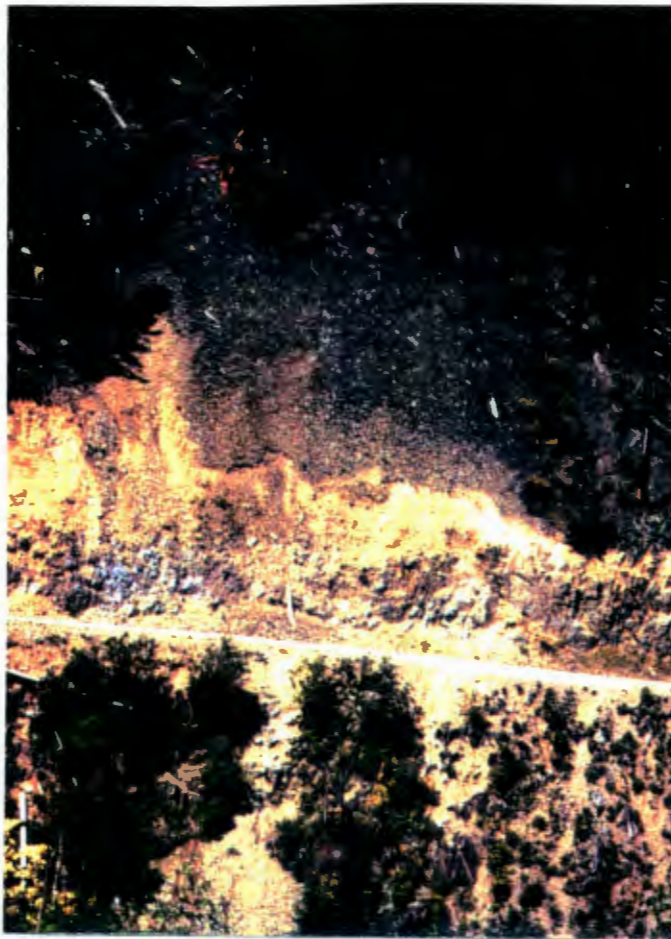
Figure 23. Effect of anthropogenic oversteepening. FS Road 37 in the NE SE 1/4 of sec 36, T.5 N. R.5 E. This roadcut has oversteepened the till and talus overlying basaltic andesite bedrock. Oversaturation has resulted in the progressive failure of the overburden which has blocked the road at times. The largest failure, on the left, is 30 m long. Note that the overburden is failing progressively uphill as highlighted by the overburden color changes.
