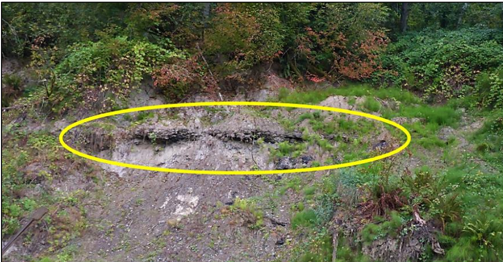
Figure 10. Example of a sample site with a log buried in sediment and exposed along a road cut (yellow oval). This log had a pre-last glacial maximum age, but was located in a post-last glacial maximum landslide deposit, indicating it had been remobilized.
