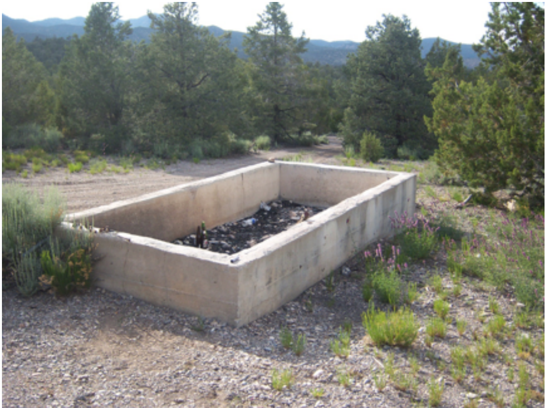
Image 16. Former cattle troughs where spring water was piped and impounded from Spring 9. Photo by USFWS
