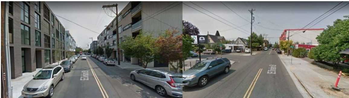
Figure 3.3 Urban collector with double yellow centerline. SE Division east of 33 rd , eastbound (left) and westbound (right) [22].
