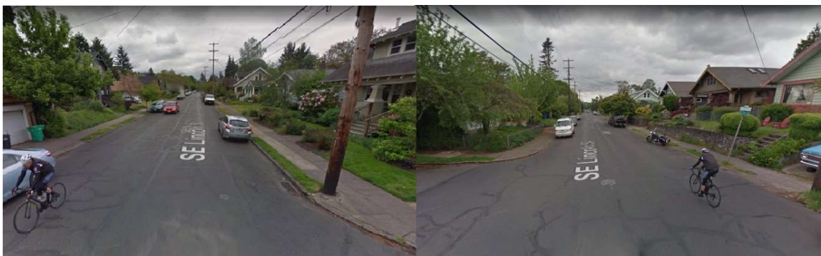
Figure 3.1 Neighborhood greenway local street without a centerline. SE Lincoln east of 48 th , eastbound (left) and westbound (right) [20].
