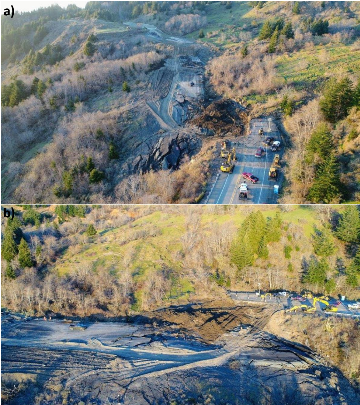
Figure 2: Drone images taken of the Hooskanaden Landslide following a recent surge in February of 2019. (a) is looking to the north, and (b) is looking to the east. Images provided by the Oregon Department of Transportation.
