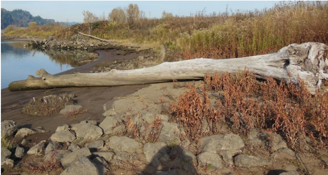
View of riprap piling at site 35MU242.
