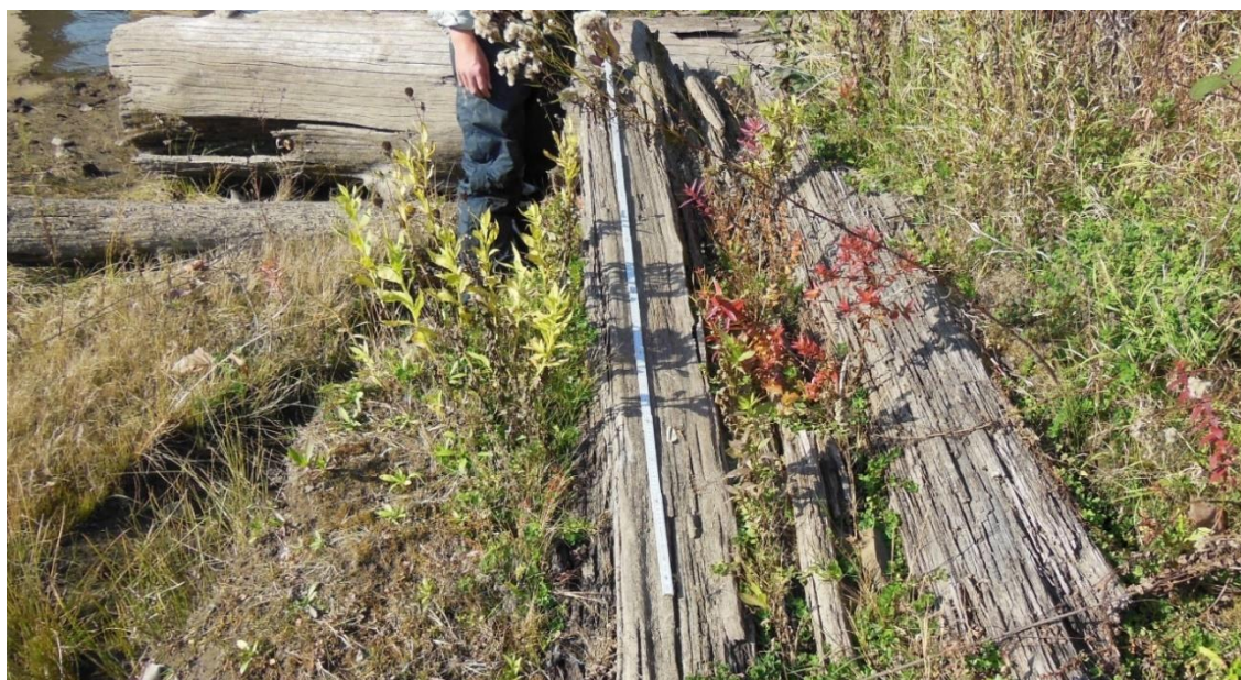
Historic dock feature at site 35MU63.
