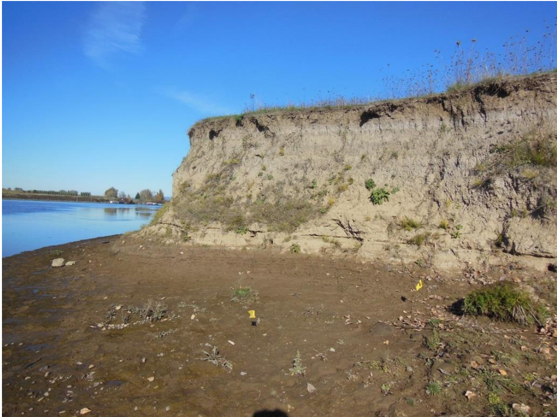
Figure 4.12. Example of sheer, exposed bank at near 90° angle, at newly identified site PJD002.
