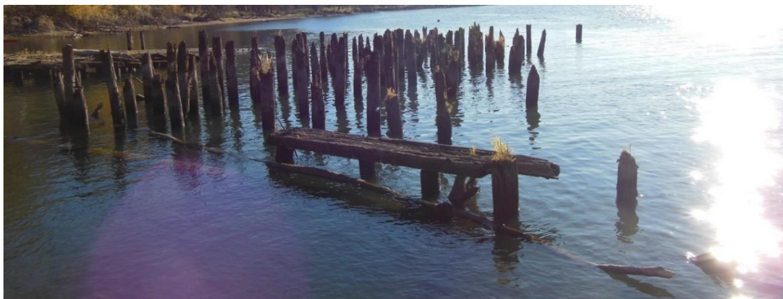
Piling field and structural elements at site 35CO66.
