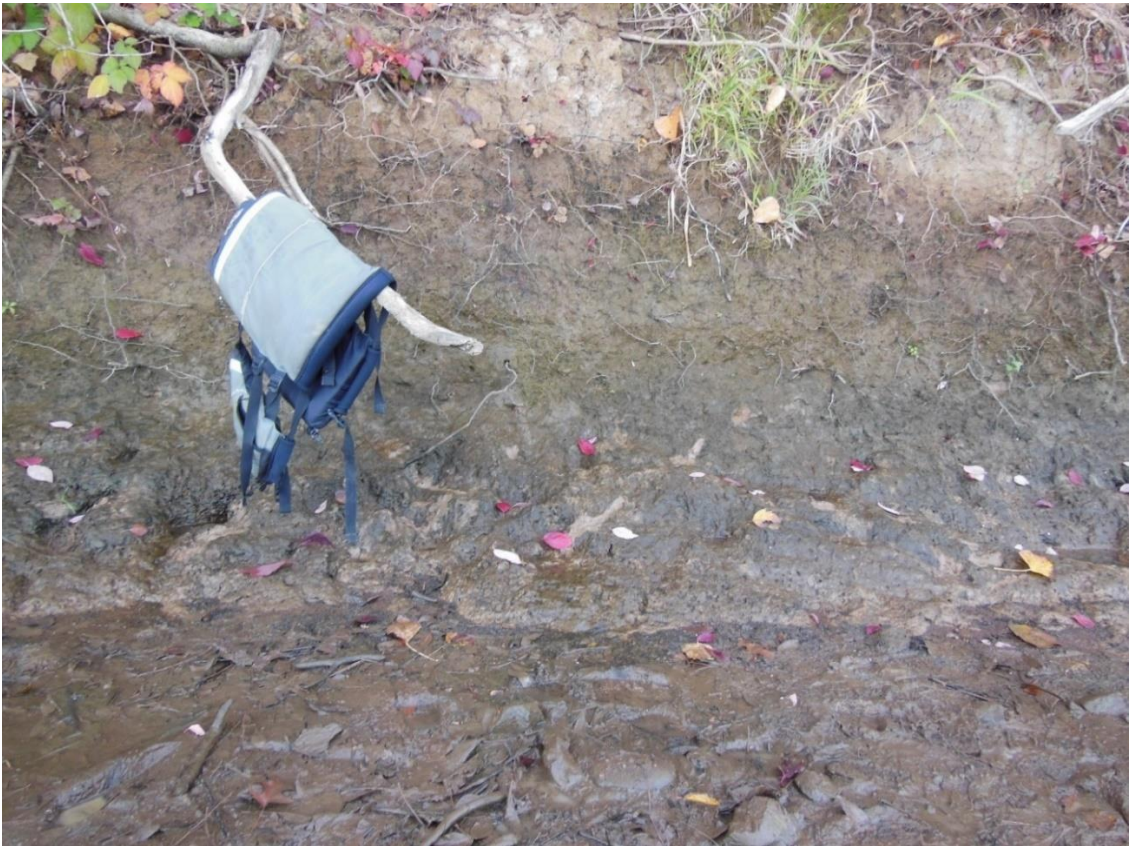
Exposed steeply angled cut-bank at site PJD006.
