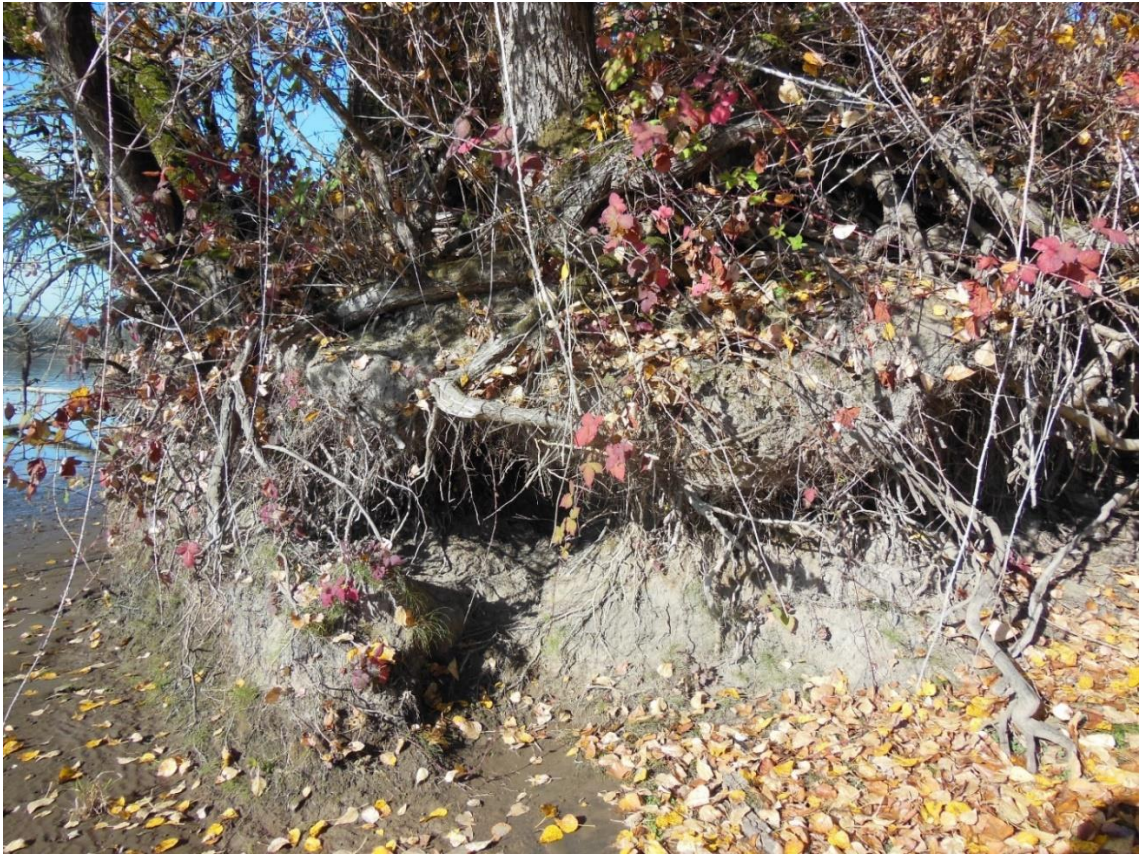
Example of undercutting.
