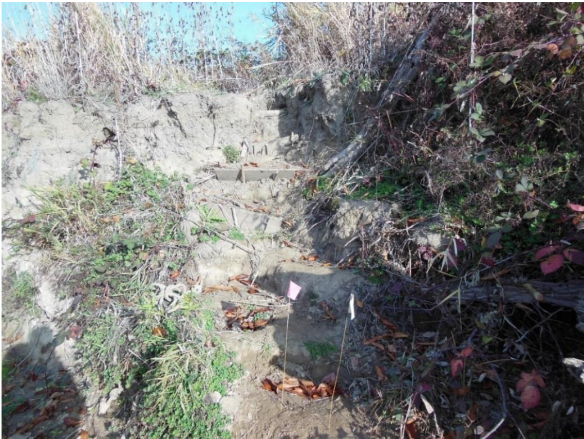
Figure 4.13. Illegally constructed trail with wood and rebar supports, leading from Sauvie Island Road to beach of site 35MU62. The trail offers easy access to multiple sites along the shoreline.
