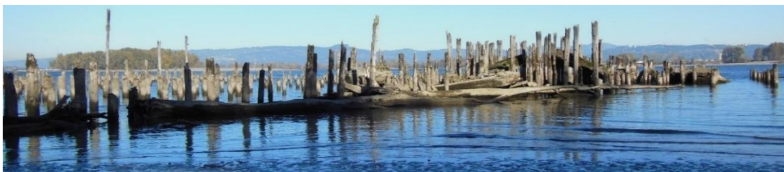
Piling field and structural elements at site 35CO66.
