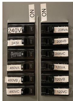
Figure 5.8: Circuit breakers of different output voltages.
