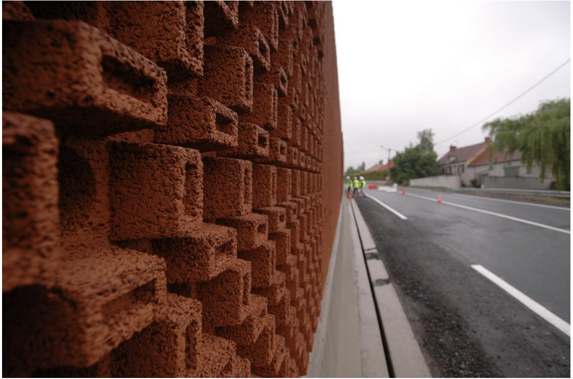
Figure 1.7: The Noise Abatement Wall [34] effectively confines noise for housing along the busy road. It contains holes ranging from 30cm to submillimeter pores because the irregular geometry makes it a bad resonator. Absorption of acoustics are strongly linked to the spectral properties of the Laplacian operator. Image retrieved from IPAM Research Articles on April 15, 2024.
