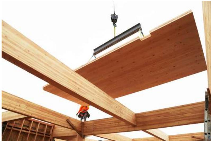
D.R. Johnson Wood Innovations located in Riddle, OR recently became the first manufacturer in the United States to receive certification from the American Plywood Association (APA) to produce cross-laminated timber. Currently, the maximum panel size that can be produced at their facility is 10 feet × 32 feet × 3, 5,
