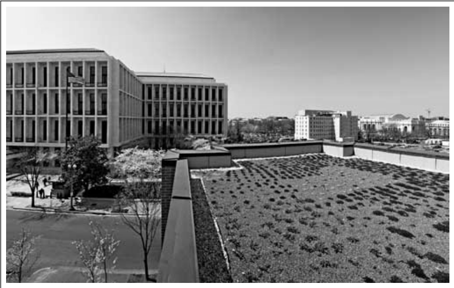
Figure 4. FCNL Building, Green Roof and Hart Senate Office Building
